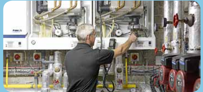
RVR Equipment being installed.
